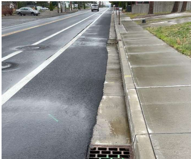
Figure 10. 2023 8th Ave. Sidewalk and Bicycle Lane Improvements (Thierman and Park Roads).
