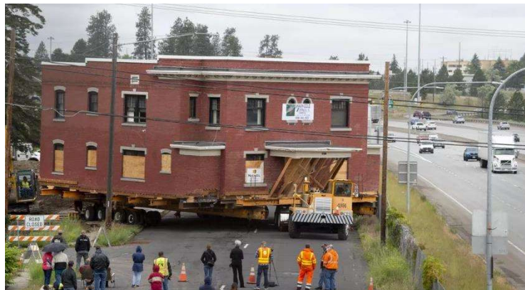
Figure 26. Rose Apartment Building. Constructed in 1910. Relocated in 2020 within East Central for affordable housing.
