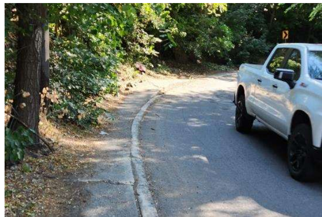
Figure 21. S. Altamont St. non-compliant sidewalk (narrow & heaved).
