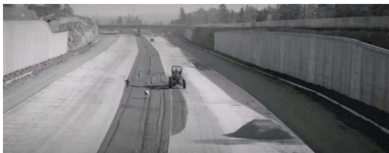
Figure 8. I-90 Construction approaching Liberty Park (from west)
