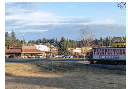
A wide highway and broad setbacks isolate development projects from their neighbors across Highway 395
