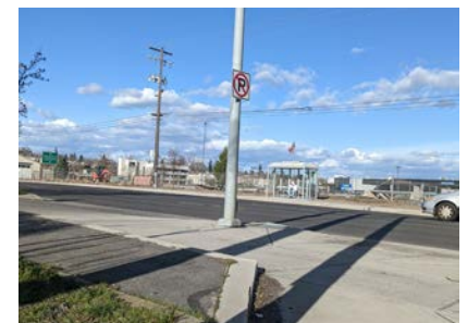
Tight quarters between traffic and transit stops decrease pedestrian safety.
