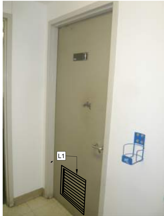
10X10 NEW MOUNTED DOOR GRILLE, TYP FOR ALL INTERIOR DOORS, SEE MECH.
