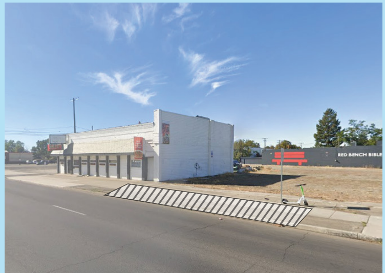
Street view of the station location, looking south (Google Street View)
