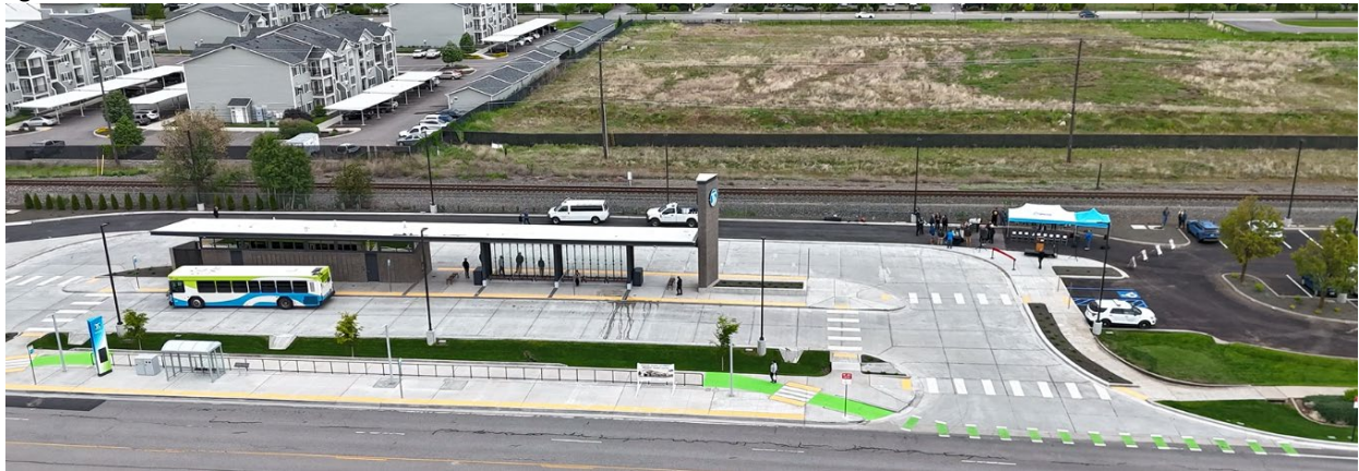
Figure 5 – Mirabeau Transit Center
